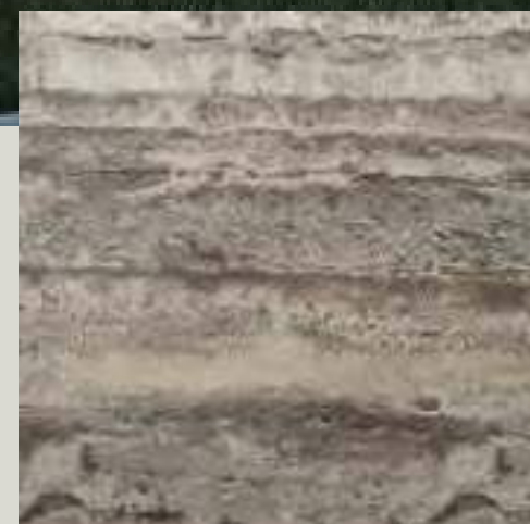
EXTERNAL FLOOR STONE
