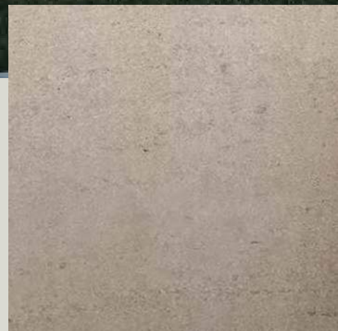
EXTERNAL FLOOR STONE
